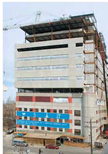
The ongoing construction of Cummings Pavilion E.
